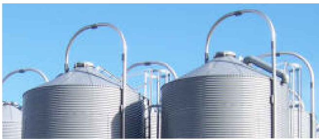
7 External Plant/ Storage Silos
